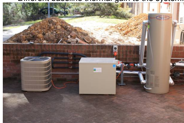
Figure 10: Location of desuperheater, compressor & buffer tank.
