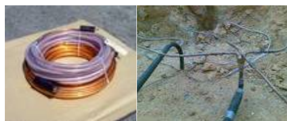
Figure 1: Copper earth loop, liquid & vapour manifold.
