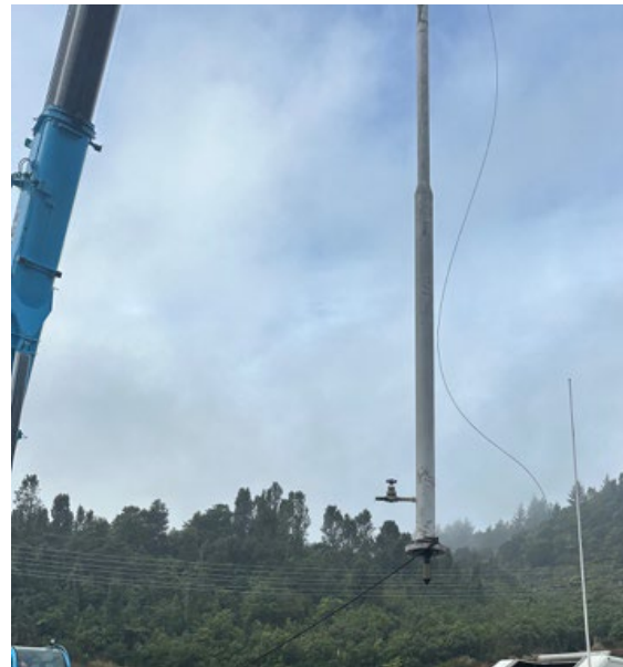
Figure 1: Successfully Retrieved CIS Tubing
