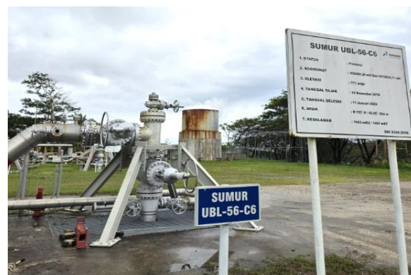
Figure 2: UBL-56 Geothermal Well.
