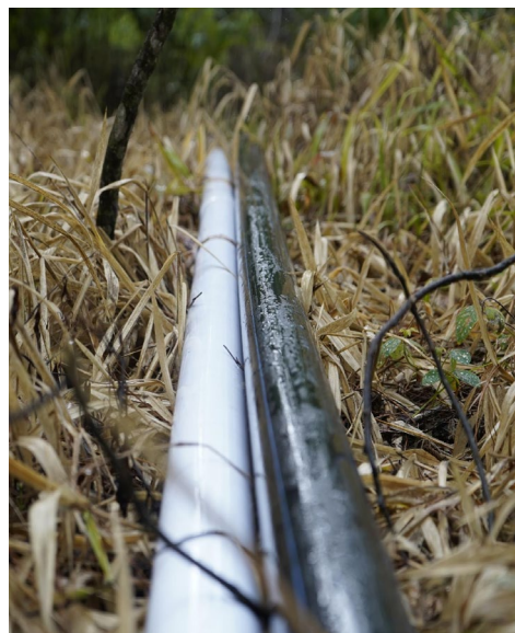
Figure 7: Use of HDPE Pipe for Agricultural and Community Water Access
